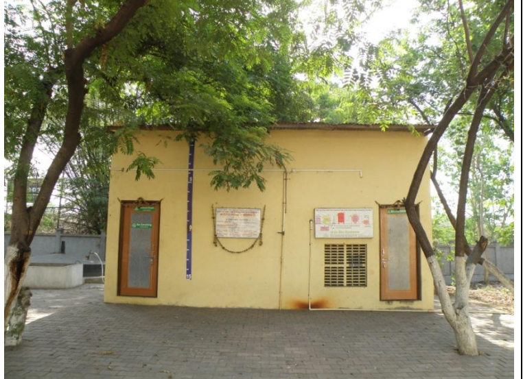
Bio Gas Electricity Generator House
